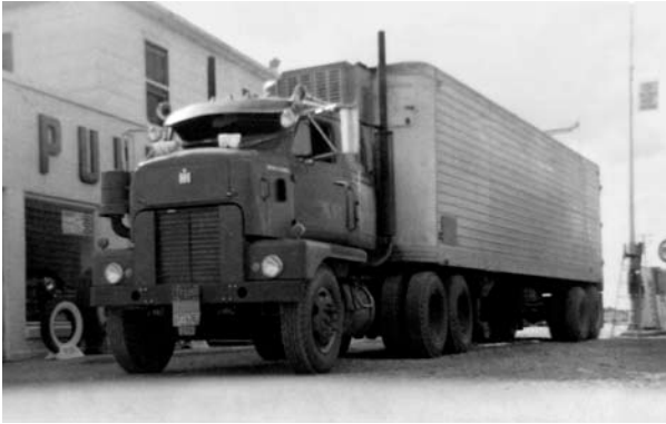
This red International RDC-405L had twin horns, spotlights, and very loud twin straight stacks. It was powered by a 220 Cummins with 10-speed Roadranger and was pulling a Brown trailer with blue Little Audrey signs. (August 1956)
