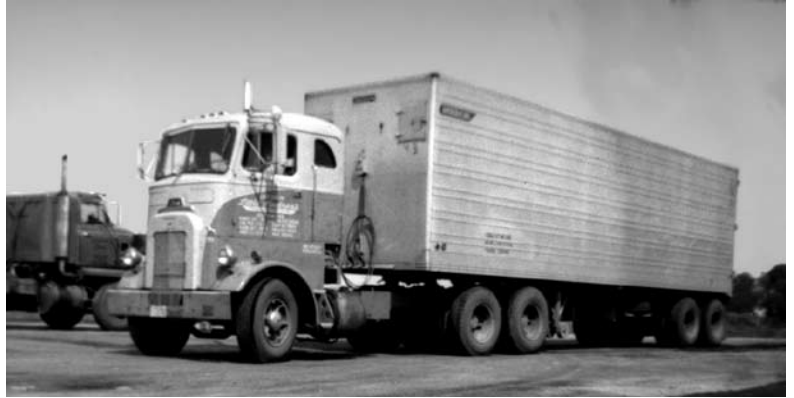
Exhibiting typical California style, this blue-and-gray Mack H-61 Cherry Picker had a long wheelbase and tag axle. But the steel spoke wheels were East Coast style. It was pulling a big, square-nose American trailer. (June 1956)
